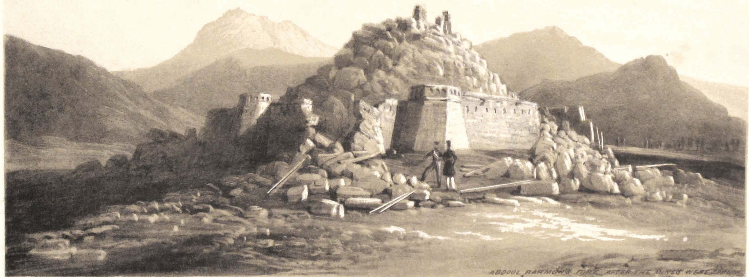
ABDOOL RAHMONS FORT AFTER THE BUNKER WERE BLOWN
